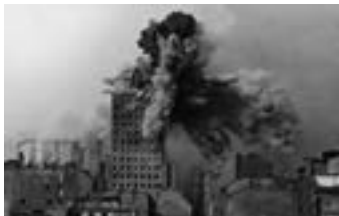
28th August 1944 - explosion from a German mortar which hit the most modern 16 story block in Warsaw. The welded structure withstood the blast. The modernist Prudential building stands to this day.
