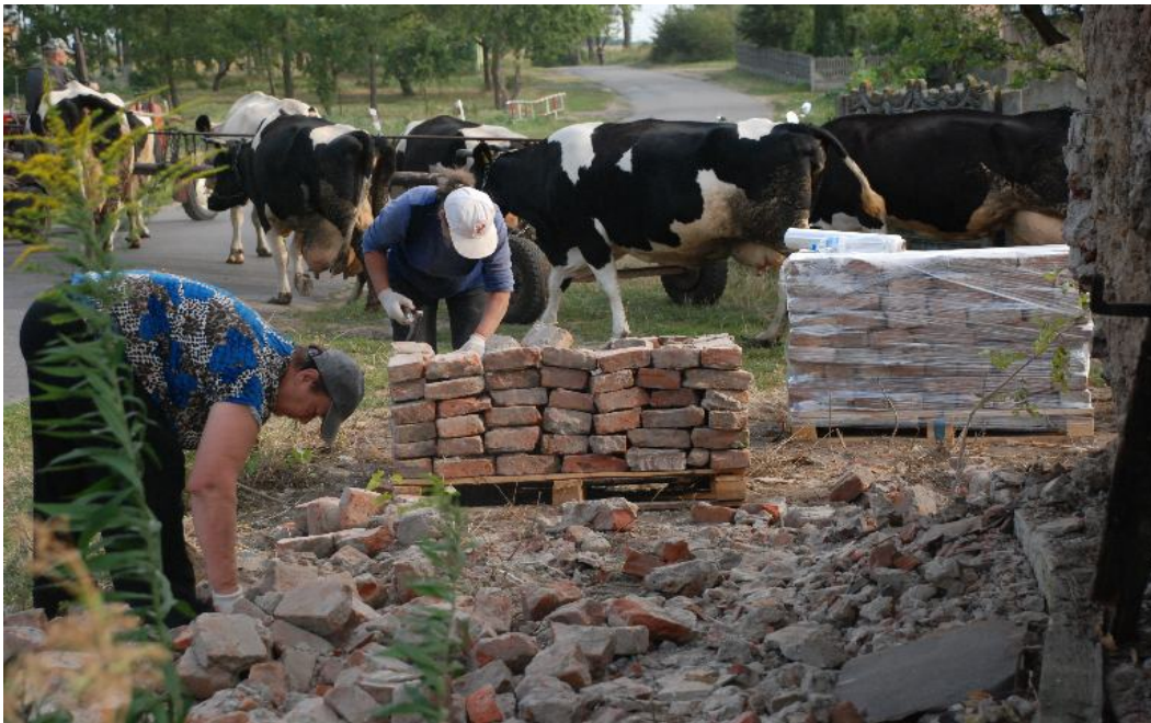
Demolition house in Kurówku, 2015
