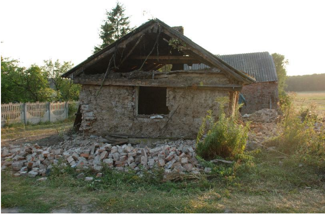
Demolition house in Kurówku, 2015
